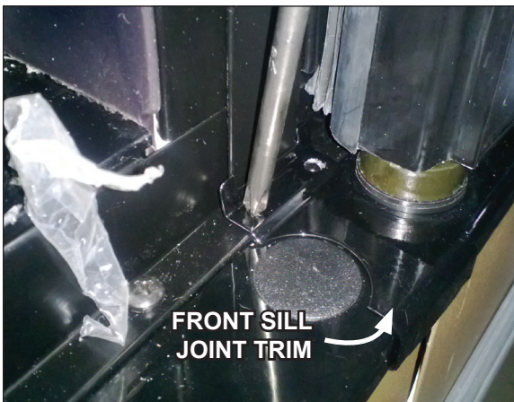
Fig. 9 Front sill joint trim
