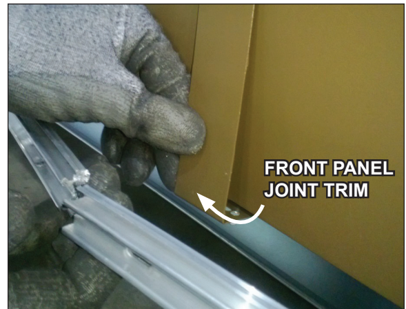
Fig. 5 Front panel joint trim
